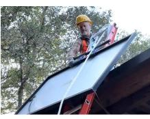
**4.** Release Break. The operator at the top releases the brake to lower the Module Handle back down to the bottom of the ladder.
